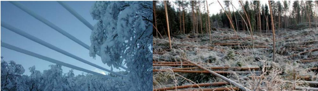
Figure 3: Snow load on power lines L-side and wind damage on R-side [4]
