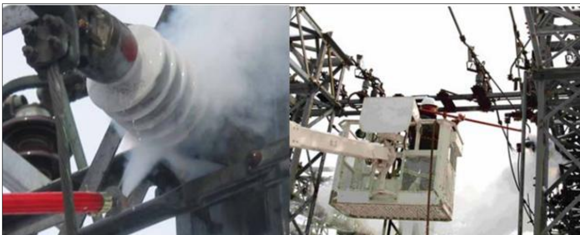
Figure 47: Steam cleaning of insulators [57]
