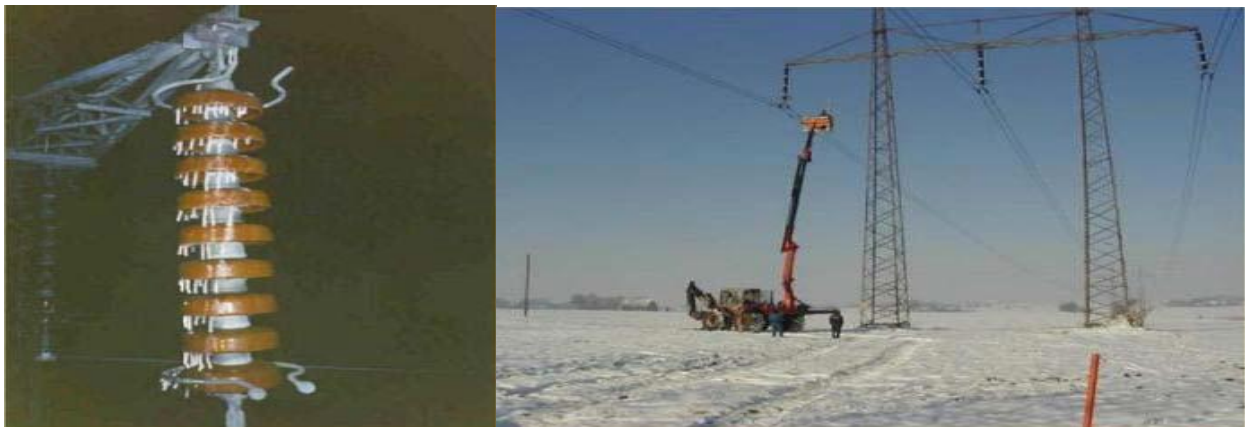
Figure 4: Icing on 130kv insulator R-side and de-icing of 400kv line L-side [6]
