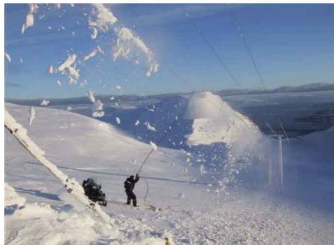
Figure 44: Mechanical method for de-icing [36]
