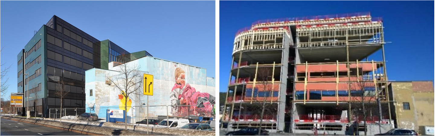
Figure 5.10: The eastern side of Solsmaragden showing the transformer close by, photos gotten from Christine Wangsnes, Union Eiendom and FUSen.no
