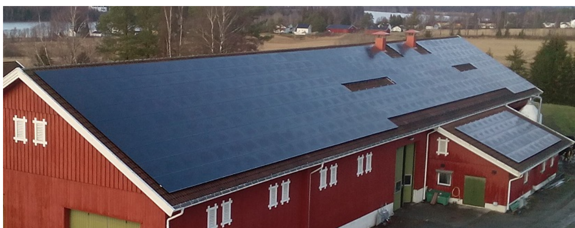
Figure 5.11: The PV system at Grøndalen Gård, photo: Karl Andreassen, Green Energy A/S
