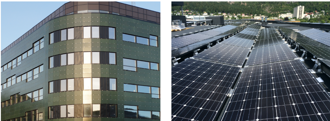
Figure 5.5: The curved western facade and roof of Solsmaragden, photos from [31]
