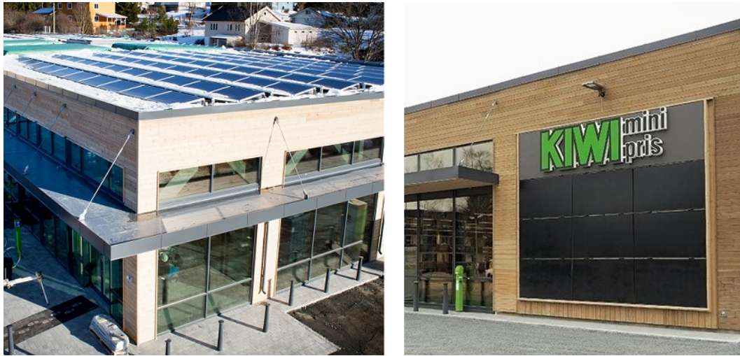
Figure 5.18: The roof and facade at Kiwi Fjeldset, photos from [37] and [38]
