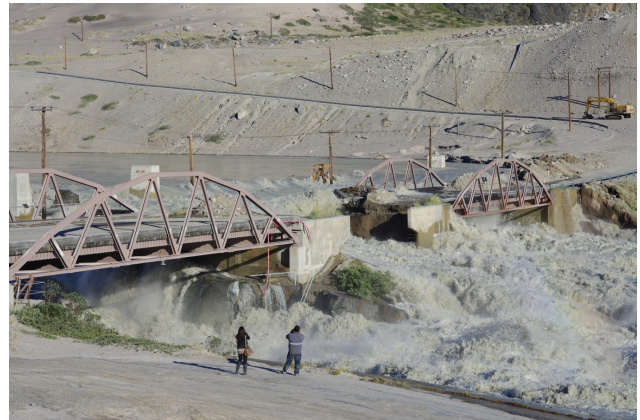
Figure 2. Photograph taken at 18:00 West Greenland Summer Time on 11 July 2012 during the flood with the Watson River Bridge being washed out. Image courtesy of Jens Christiansson.
