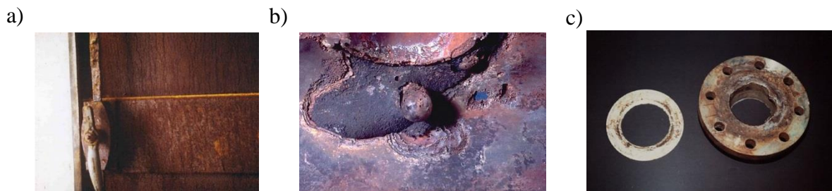
Figure 6 - Example of a) uniform corrosion; b) galvanic corrosion and c) crevice corrosion (16)
