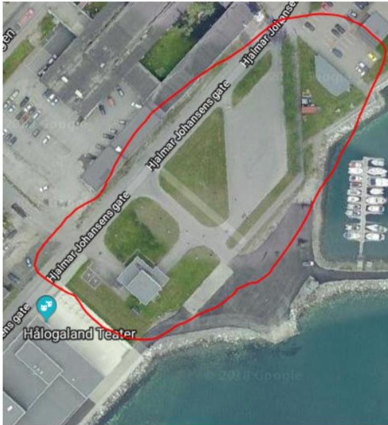
Figure 3.1: Storage area for BTES system for Kvitebjørn.
