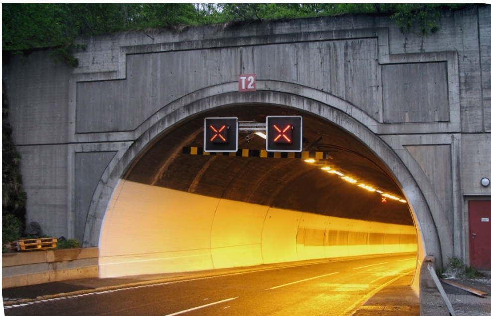
Figure 3: Picture showing the entrance for the Tromsøysundtunnelen in Tromsø, Norway.
