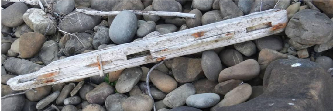
Figure 2. Japanese tsunami marine debris wooden beam showing mortise and tenon (post and beam) carpentry (JTMD-BF-248). Photo by NC Treneman.
