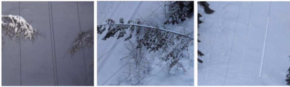
Fig. 1. Common faults on power lines (from left to right): trees growing too close to power lines, trees lying across power lines, icing on power lines. In warm countries, icing on power lines may not be a relevant fault; however, in cold countries, such as Norway, it is a very serious problem since thick icing accumulated on power lines can cause a great deal of damage to the lines.
