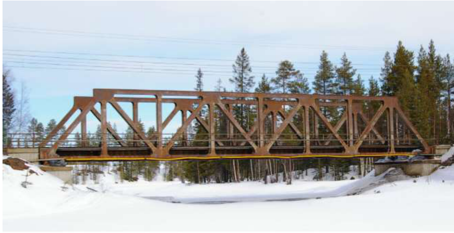
Figure 2: Steel truss bridge over Åby River, built 1955
