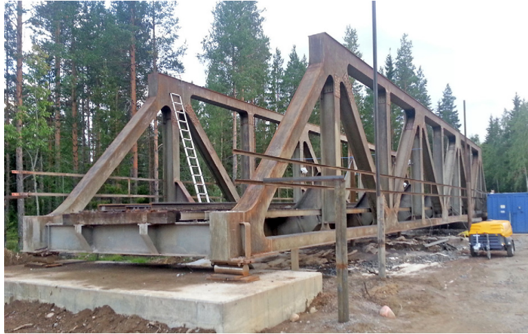
Figure 4: The bridge placed on new temporary supports.
