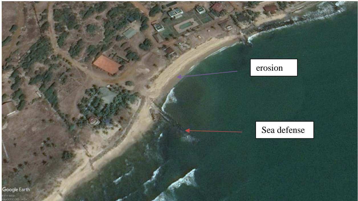
Figure 17. Example of sea defense structure across the direction of sediment transport showing erosion behind it. Direction is from left to right. Source: Google Earth, 2020
