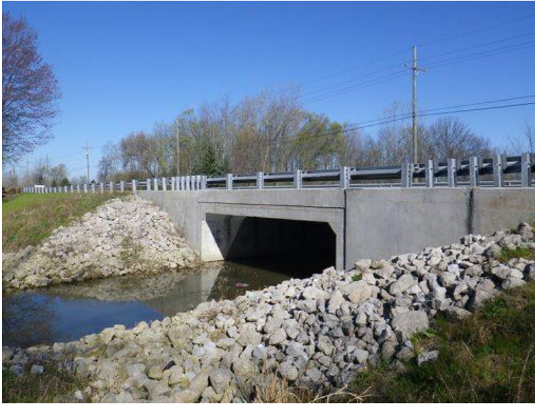
Figure 2-16: Example of a culvert bridge (Northwest Consultants, 2019).
