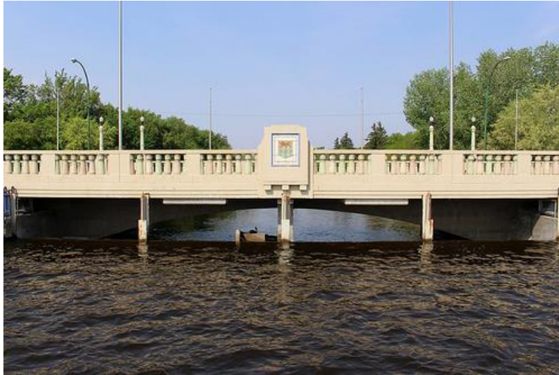
Figure 2-7: Albert Memorial Bridge as an example of beam bridge (Historic Albert Memorial Bridge, 2015).
