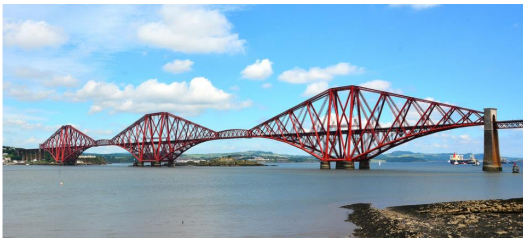
Figure 2-11: The forth bridge as an example of cantilever bridges (McBey, 2015).
