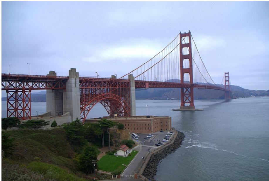
Figure 2-12: Golden gate bridge as an example of suspension bridges (Bierman, 2017).
