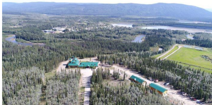
Figure 2 - First Nation of Na-cho Nyäk Dun administration building on the corner of C6 site, overlooking Village of Mayo. First Nation of Na-cho Nyäk Dun Facebook page.
