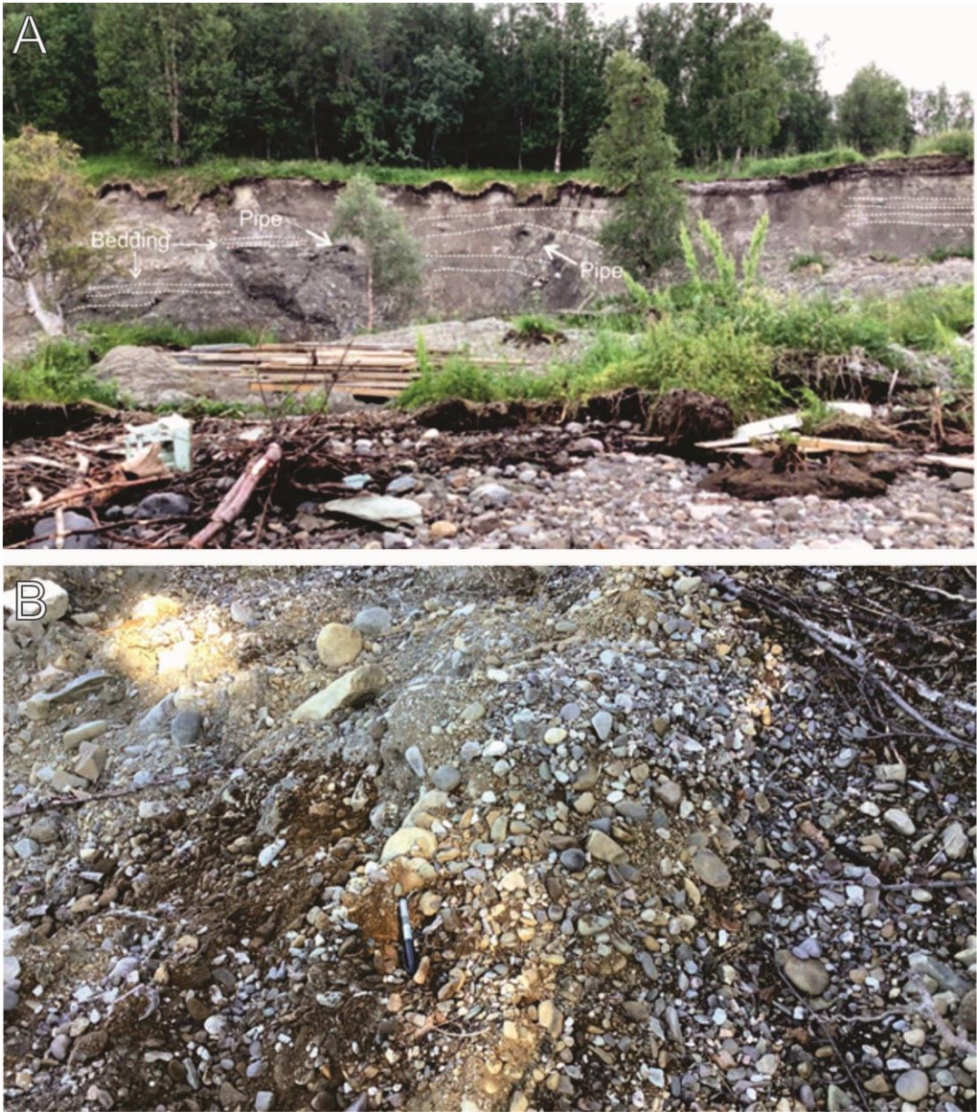
Figure 45 A) Back scarp with exposed bedding (white-dashed lines) and soil pipe structures. Vegetation and debris deposited below scarp. B) Landslide debris.
