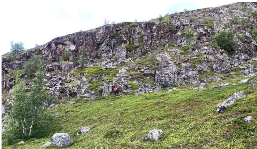
Figure 58 Fractured bedrock at Storhaugen, east of section C.
