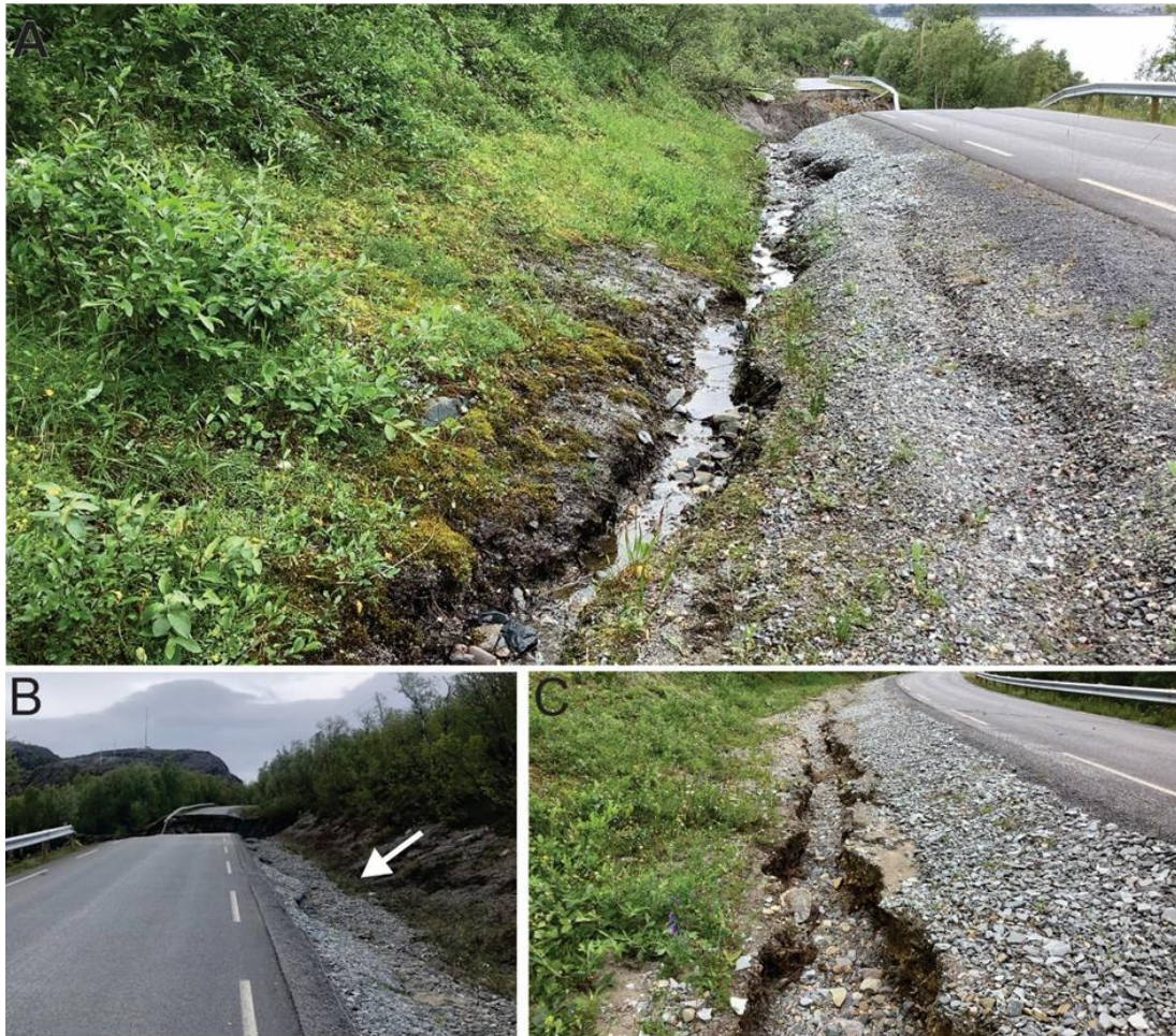
Figure 85 Eroded channels in the ditch system along the Kråknesroad north of the section B. B) Dry channels in the ditch south of section B. C) Close-up of dry channels.
