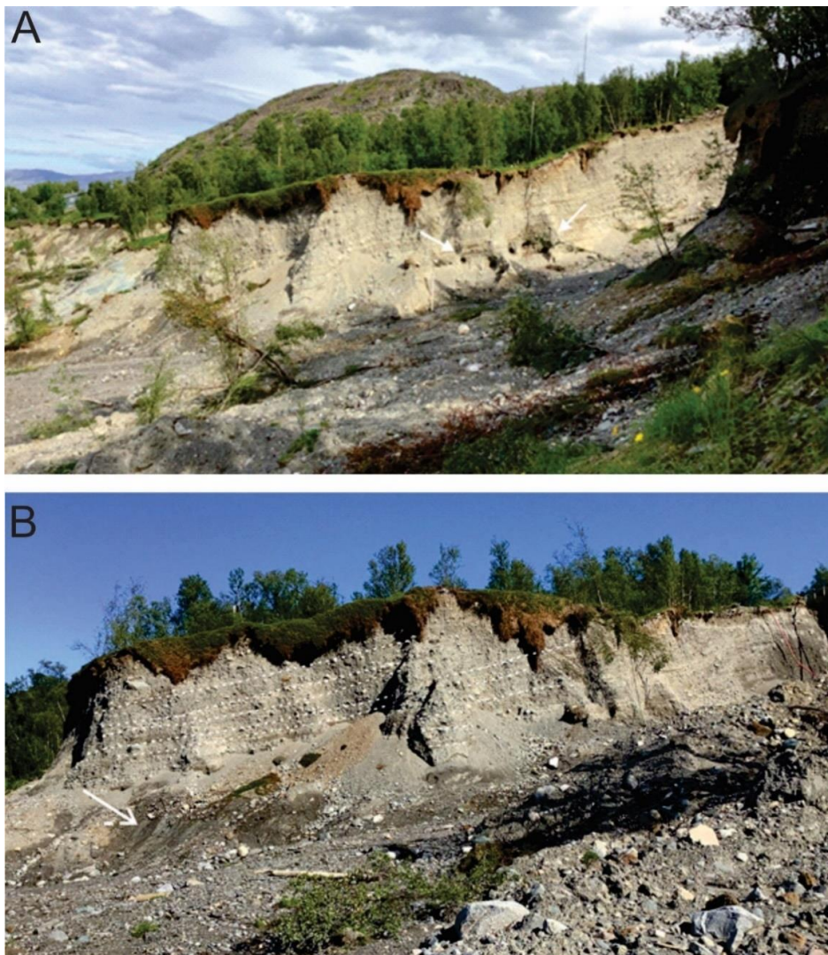
Figure 51 A) Back scarp in outcrop 8. Arrows point at soil pipes within the back scarp. B) Beddings of material 6. Arrow points at beddings of clay/silt.
