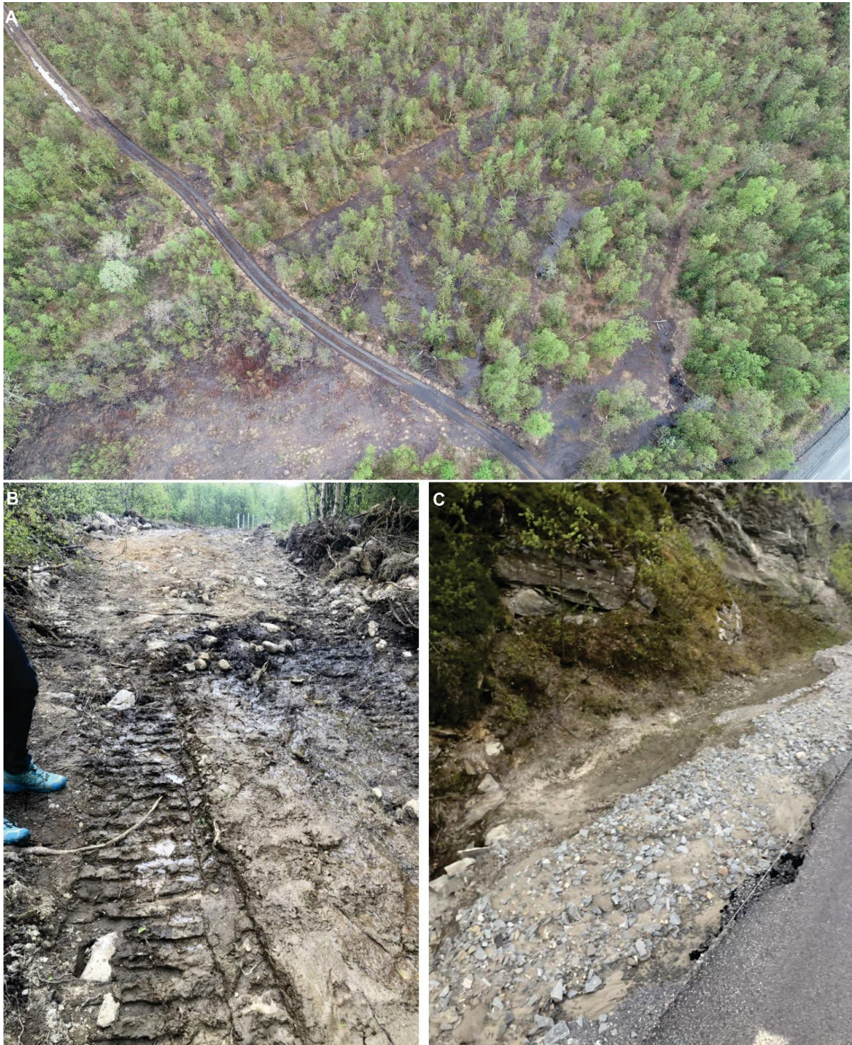
Figure 84 A) Wet area in Kråknesdalen above the Kråknes Road on June 7 th , 2020(Photo courtesy of Anders Bjordal, NVE). B) Moist tractor road on July 28 th , 2020. C) Erosion from water streams in the ditch along Kråknes Road on July 28 th , 2020.
