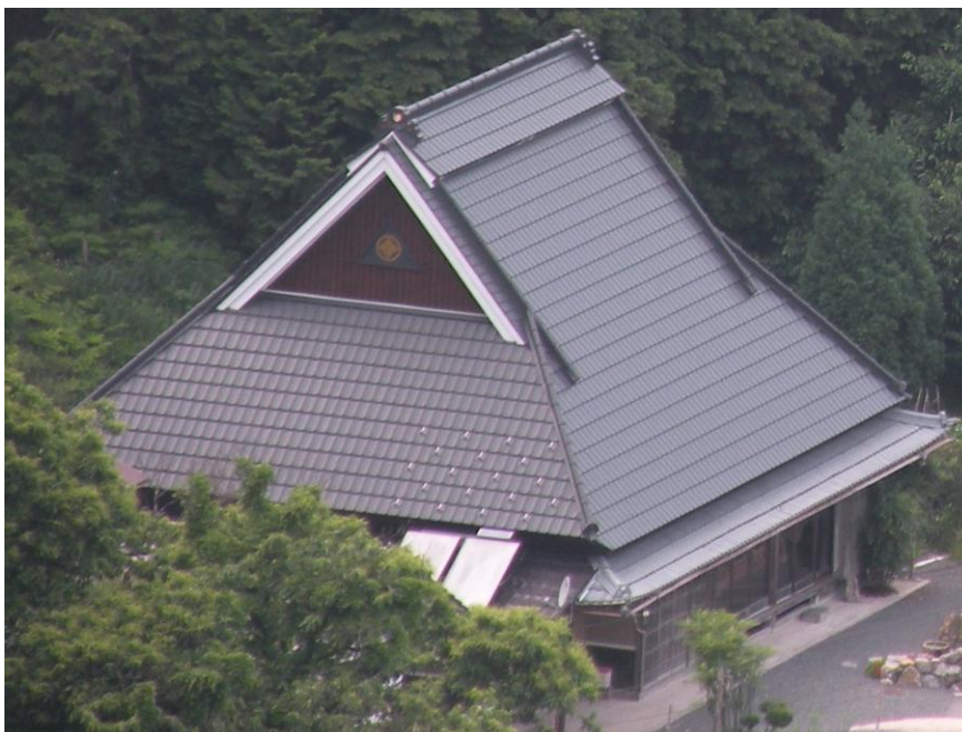
Figure 5.3 thatched roof covered by tin which imitates traditional tiled roof
