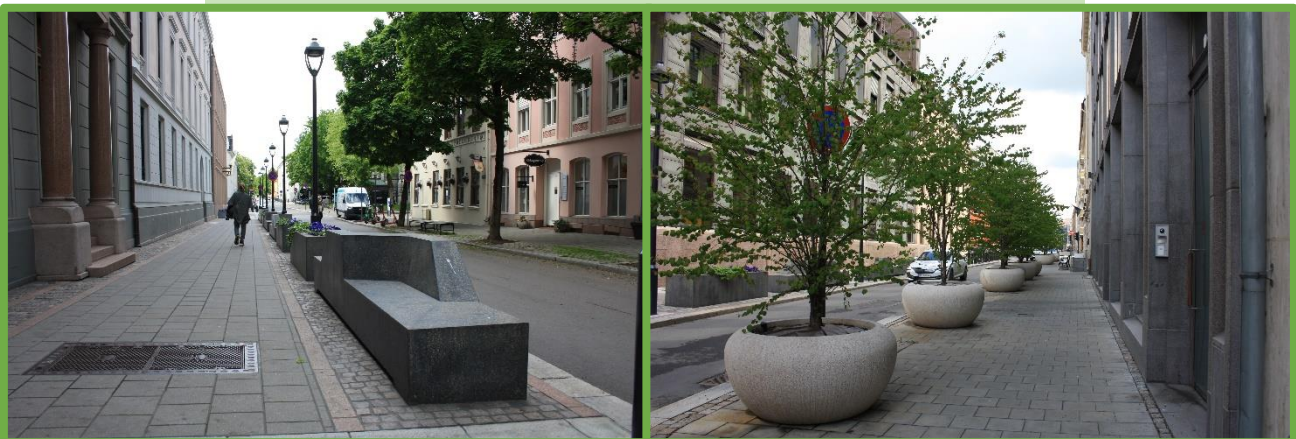
Pictures 22 & 23 33 – Integrated security measures around Kvadraturen.
