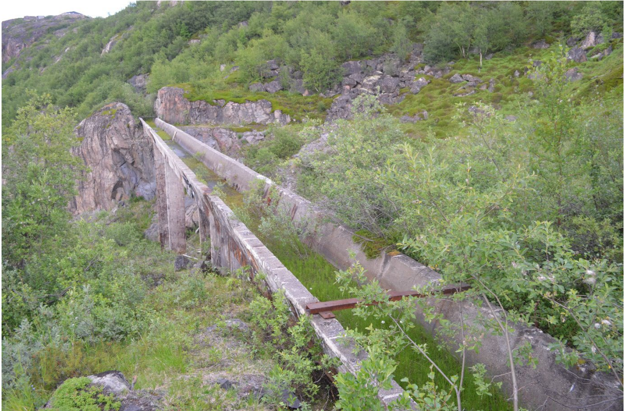
FIGURE 5. 1960s concrete mine tailings tunnel at Sydvaranger (July 2020, photograph by author).
