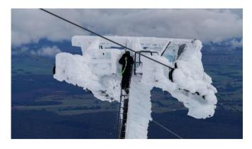
Figure 2. Ice on Gondola support tower, Mt Ruapehu [14]
