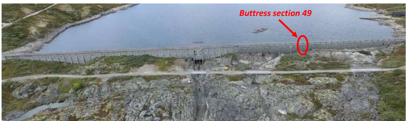
Figure 1. Photograph of dam over Kalhovdfjorden with buttress 49 marked in red
