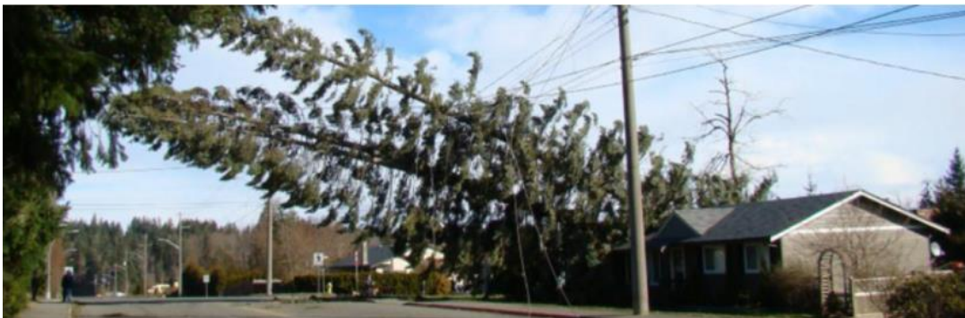
Figure 8: Example of tree lying across power lines.
