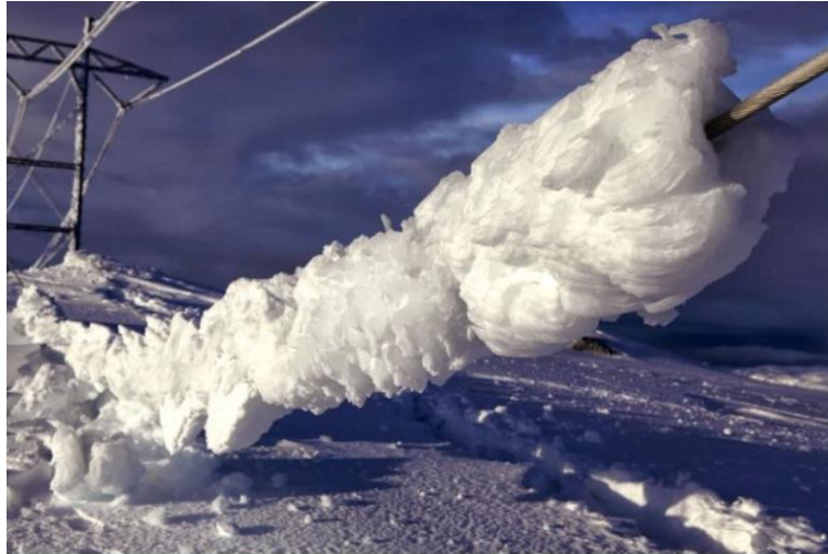
Figure 9: Extreme case of icing on power lines
