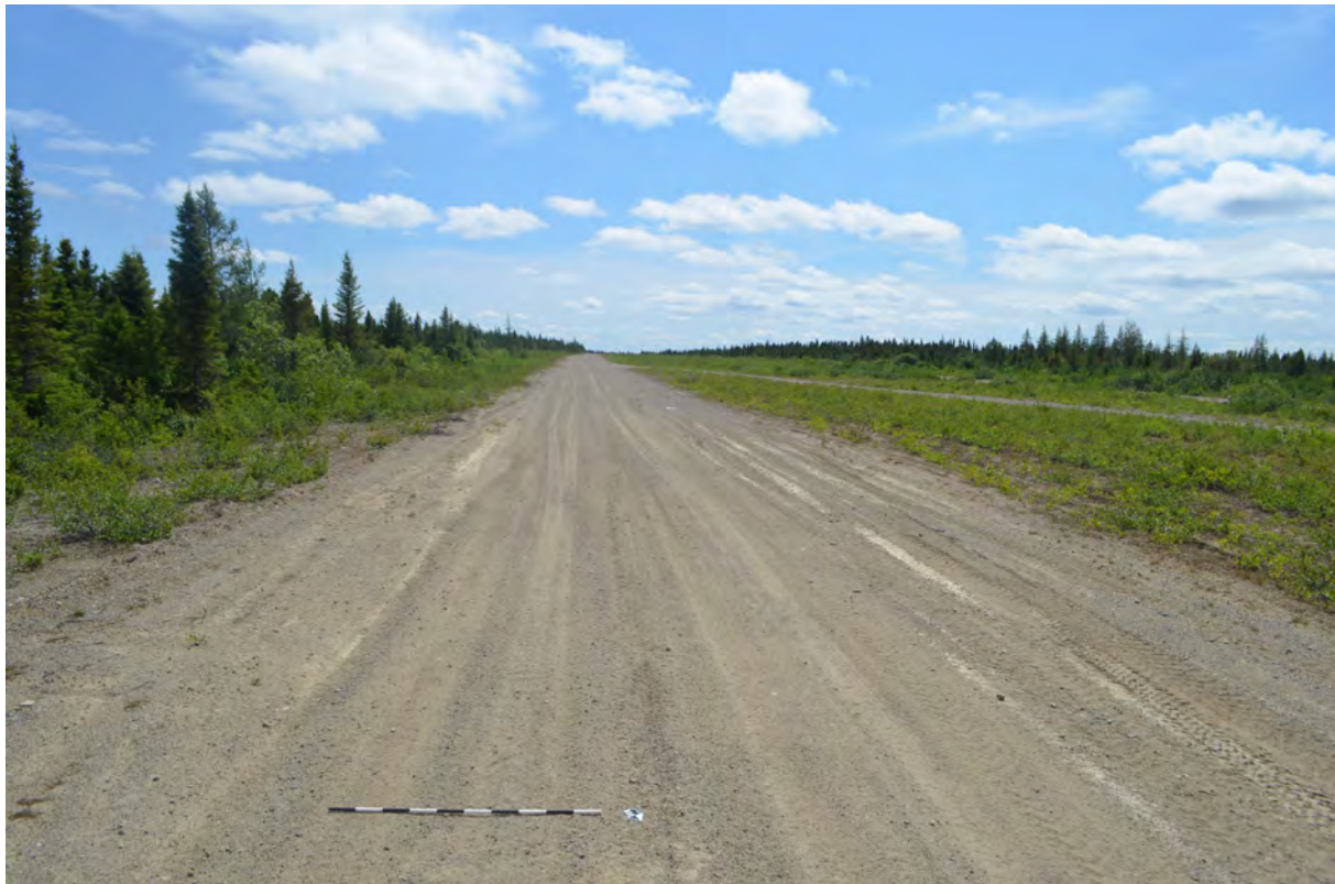
Figure 31: Airstrip at Ashuanipi River near Ross Bay Junction, Labrador used approximately from 1957 to 1959, July 15, 2021. Stadia rod and north arrow to scale.
