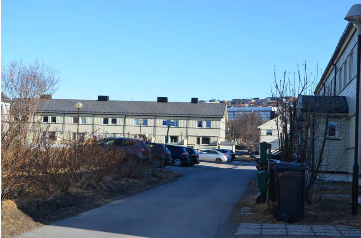
Figure 50: Expanded car parking behind post-war workers' row houses, May 10, 2021.
