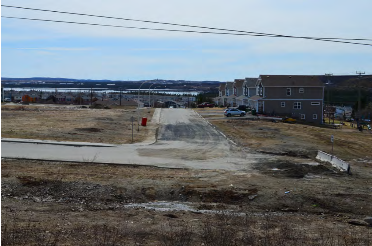
Figure 62: Unfinished subdivision in Labrador City, May 24, 2019.
