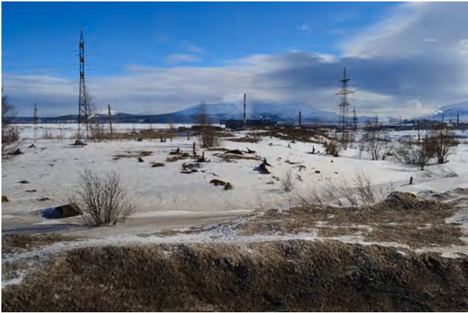
Fig. 7. Severonickel plant from E105. The southern suburb on Monchegorsk, made up of 1970s and 80's nine-storey panel block apartments is barely visible along the horizon on the left hand side of the picture (photo by the author).
