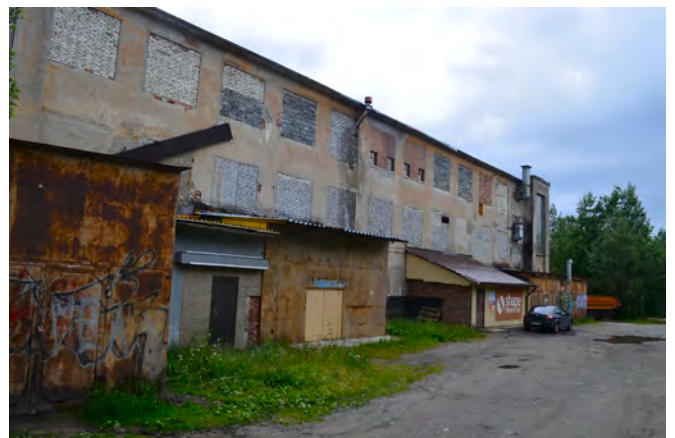
Figs. 10. Shop inside of a retrofitted Khrushchev-period building with bricked-up windows and built-on attachments - back side (photos by the author).
