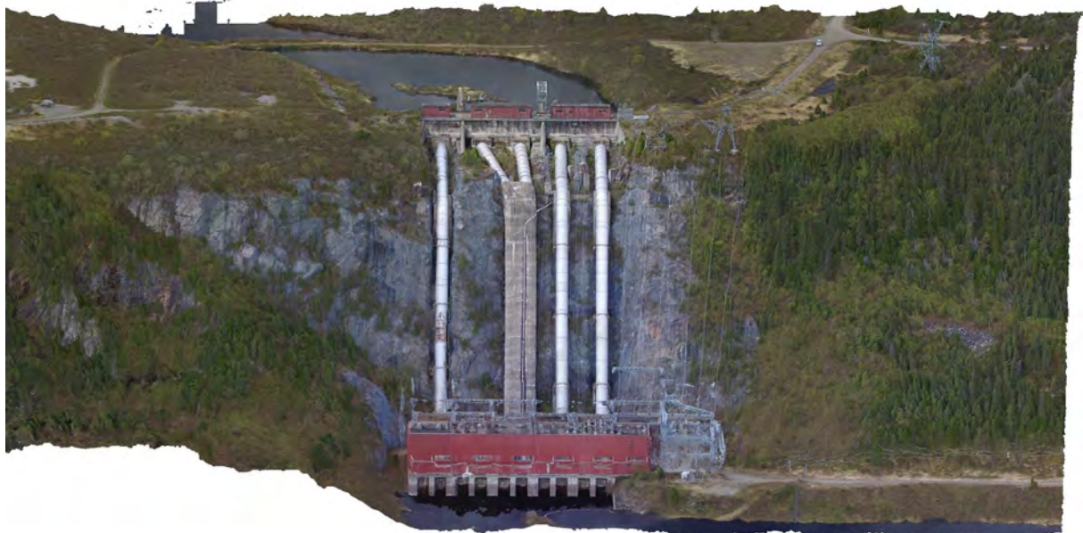
Figure 32: Drone orthomosaic profile of the Twin Falls hydroelectric power plant – power house below, penstocks in the middle, intake station at the top, and power canal above that. Image compiled by James Williamson.
