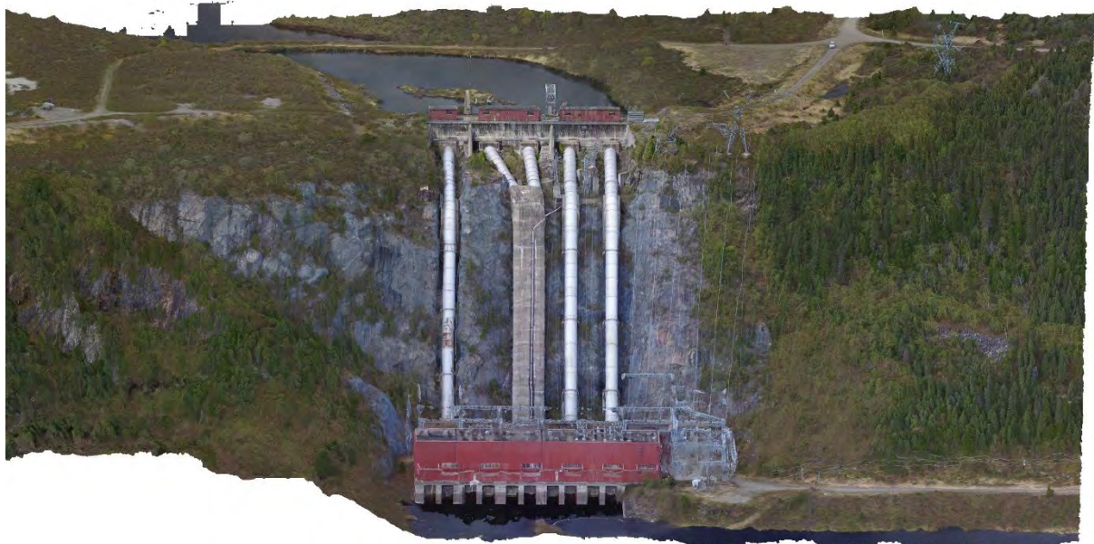
Figure 11: Drone mosaic of the intake station, penstocks, and powerhouse (image by James Williamson).
