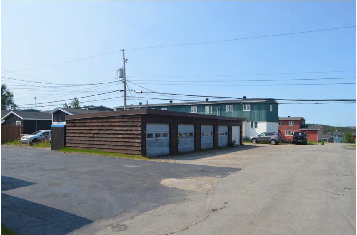
Figure 58: An original 1960s garage in Wabush with original cedar plank siding that matched many of the original homes, July 13, 2021.
