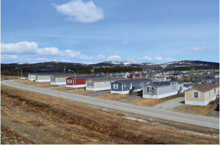
Figure 11.2 — Trailer home subdivision, Labrador City, Labrador, an example of fast-built modernity. (Photograph by Anatolijs Venovcevs).
