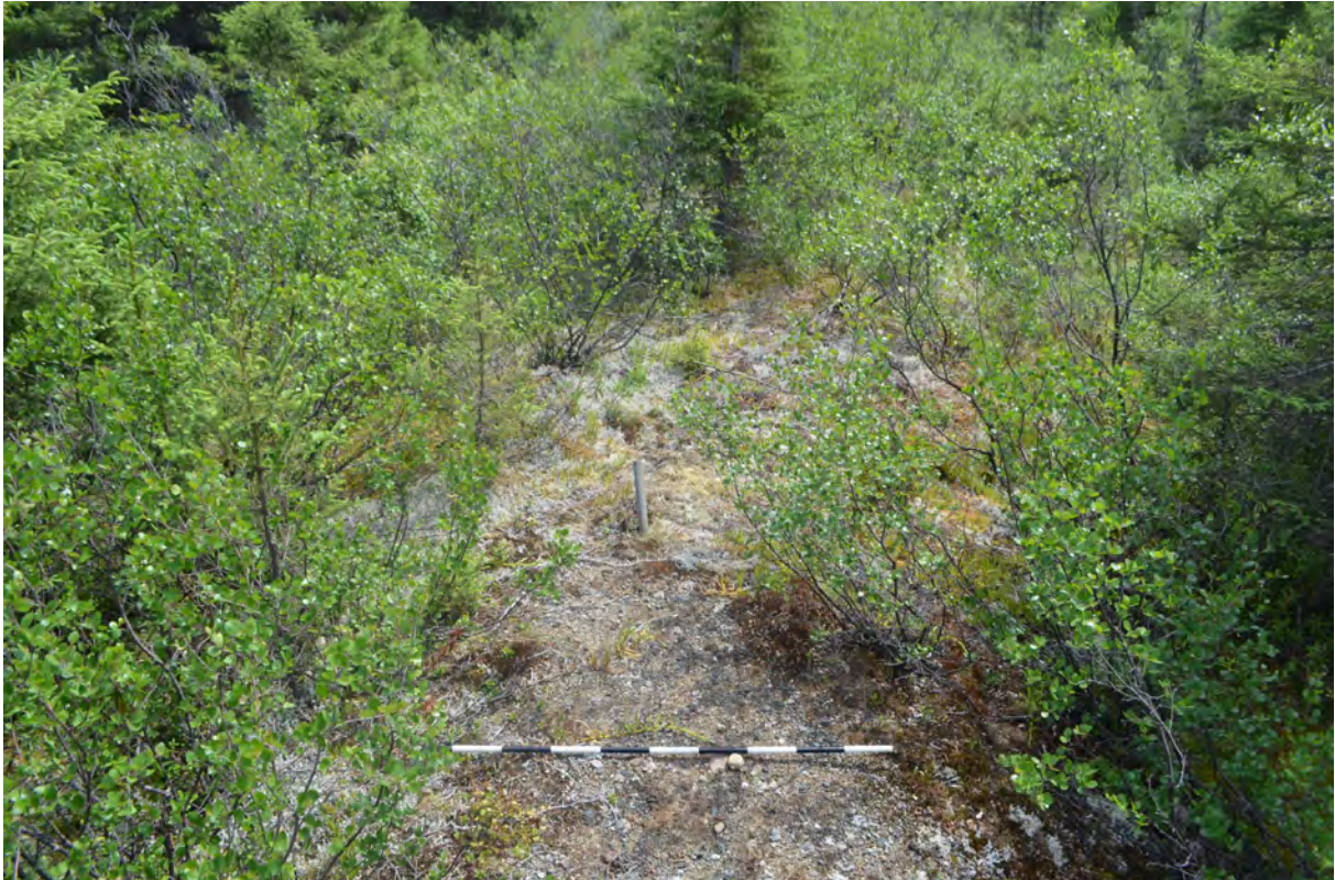
Figure 86: Alders growing over a buried water line at a former camp at the Ashuanipi runway site, July 15, 2021.
