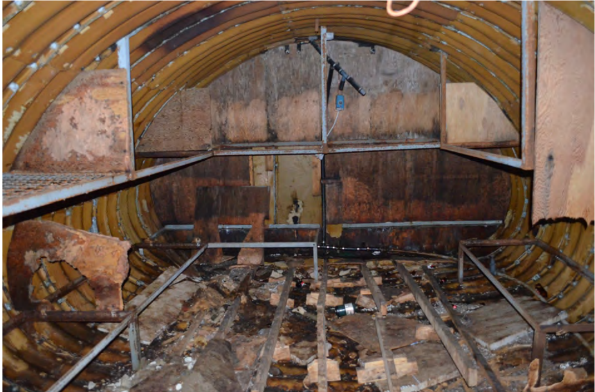
Figure 77: Cold War-era bunker in western Labrador, August 18, 2019.
