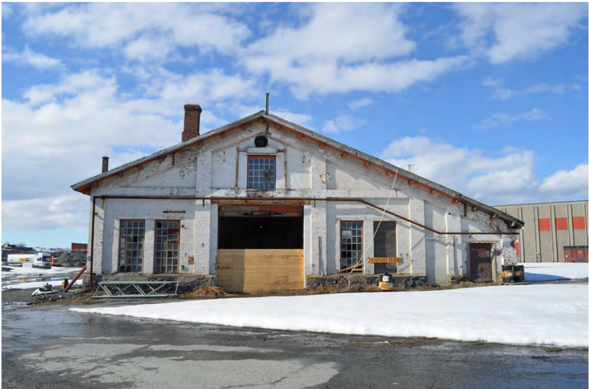
Figure 36: Photography recalling moments of encounters with things, old machine workshop Sydvaranger mine Bjørnevatn, May 9, 2021.
