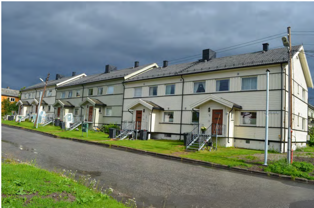
Figure 45: Workers' houses in Kirkenes, July 18, 2020. These are designed as a cultural environment of national interest and are offered some degree of protection in the municipal plan.
