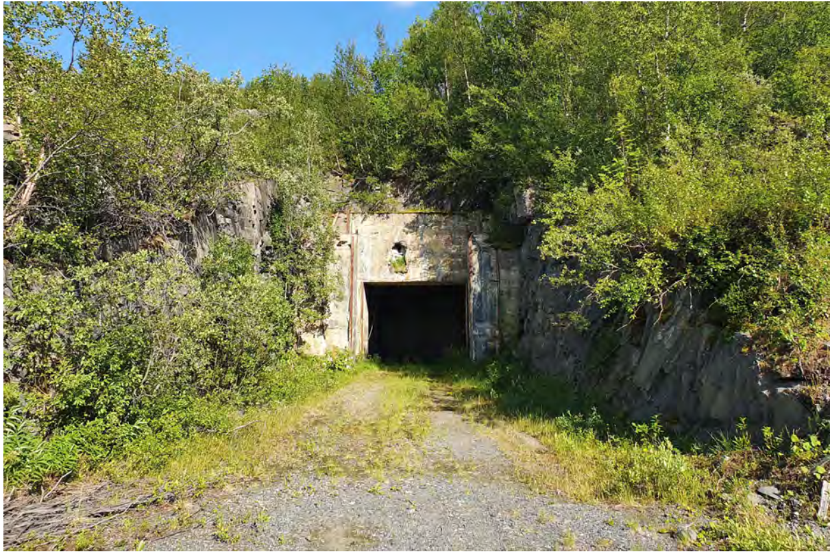
Figure 79: Tunnel inside the Sydvaranger mine, July 25, 2020. This is adjacent to the famous 1944 tunnel where much of the Kirkenes and Bjørnevatn population hid during the liberation of the area. This lesser acknowledged tunnel, originally for storage, was reinforced with concrete in the event of a future war. Thus, it is another marker that the mine continued to be seen as a vital place for protecting the local population.
