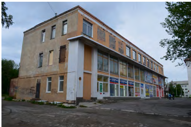
Fig. 11. Shop inside of a retrofitted Khrushchev-period building with bricked-up windows and built-on attachments - front side (photos by the author).
