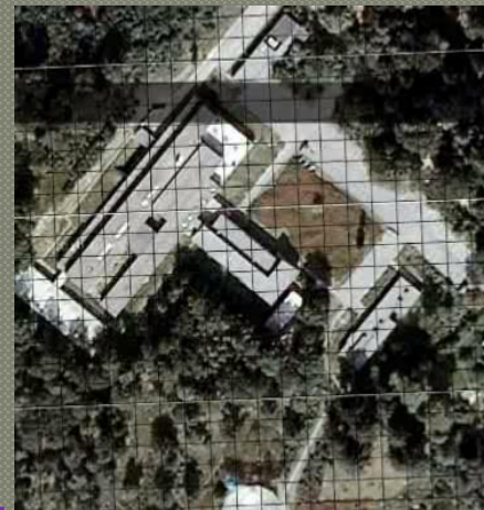
Control Centre (Dwingeloo)
