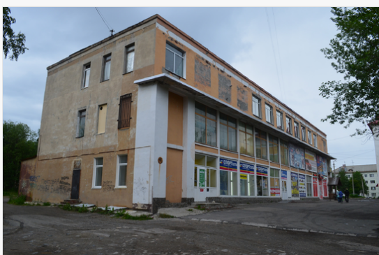
Shop inside of a walled-up, built-on, and retrofitted Khrushchev-period building with bricked-up windows and built-on attachments - front side (photos by the author).
