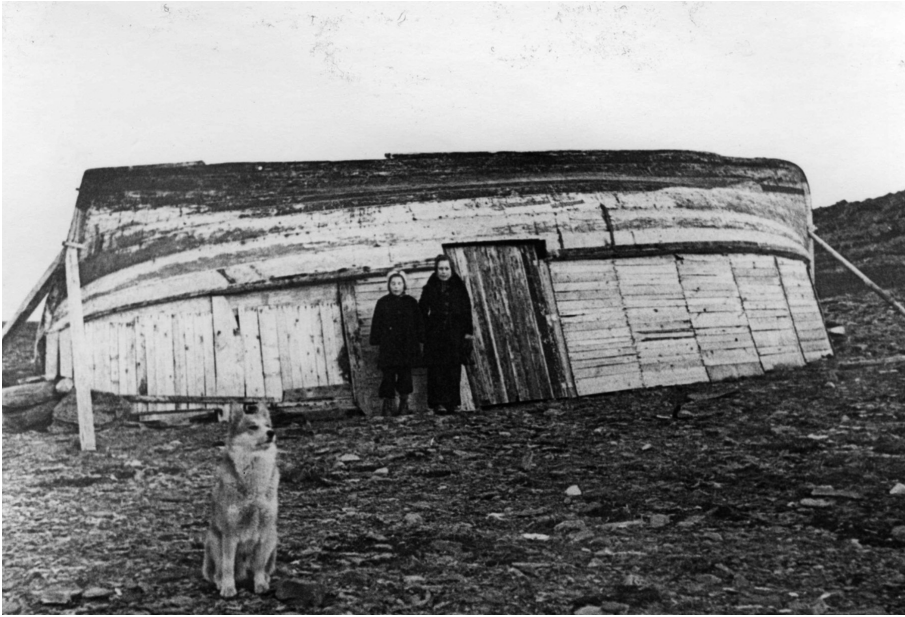
Fig. 16.2 Northland boat turned dwelling for homeless natives in the village of Gamvik, Arctic Norway, after the German retreat in November 1944 (photo: The museums for coastal heritage and reconstruction in Finnmark).
