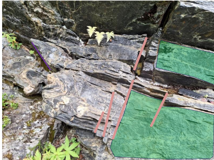
Figure 35 Joint set 1 (orange) & 2 (green) at location 7
