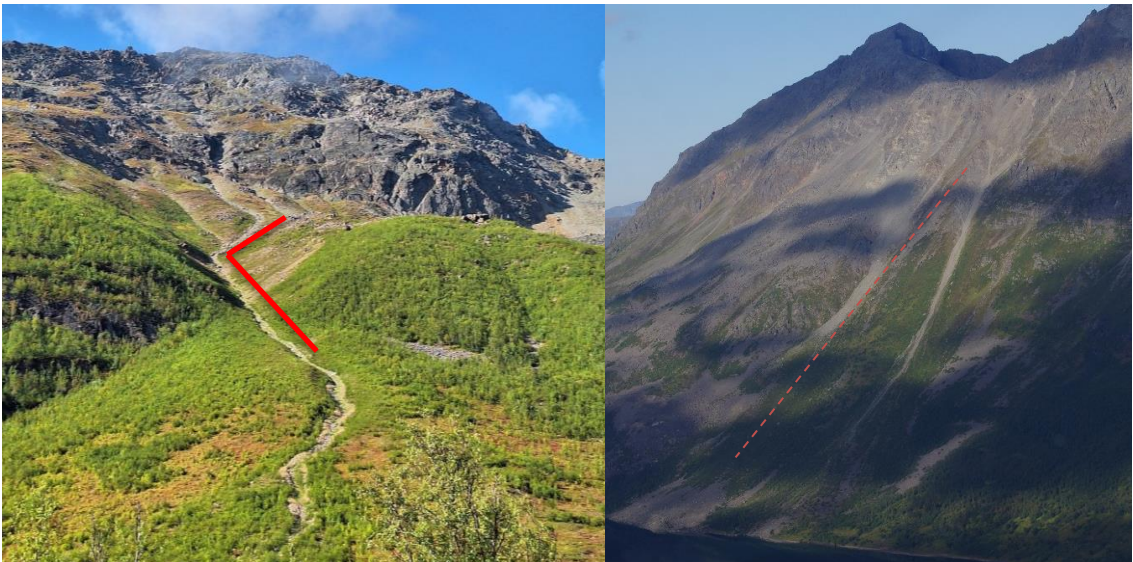
Figure 31 Southern (left) & northern (right) lateral boundary (red; inferred limit: dotted line) with debris flow tracks (Photo to the left taken by NGU 2019)
