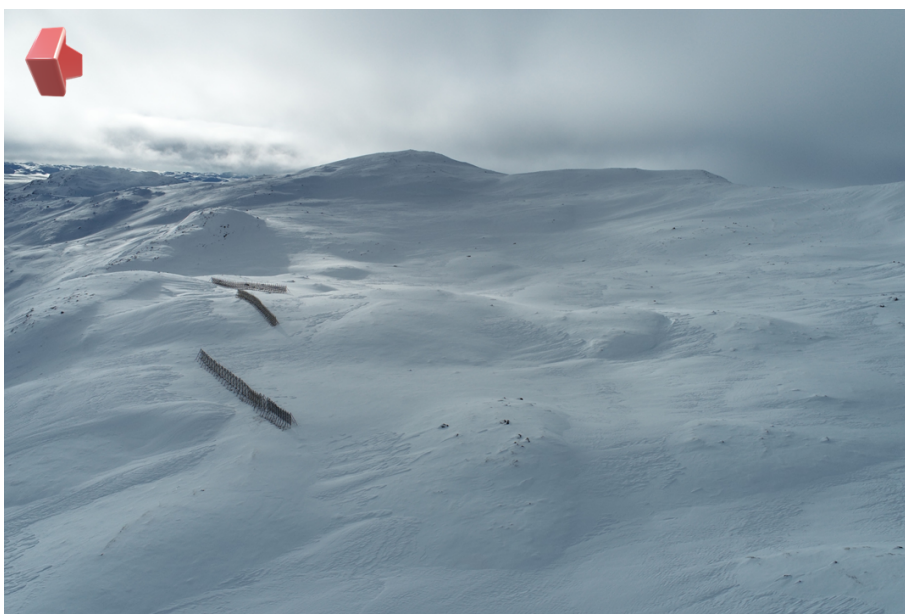
Figure 3.1.5: The snowdrift catchment plateau above avalanche towers Støl 1 & 2. Direction of picture towards south. Patches of windslabs on top of the general snow cover (wind crust) can be seen. Picture taken by Solbakken, E. 21.02.2023. Red arrow indicates north direction.
