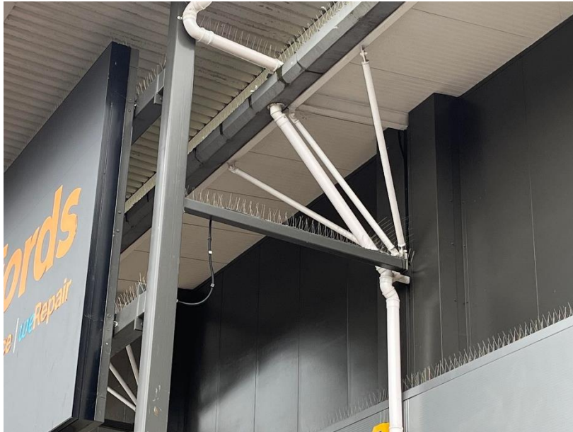
Figure 10: Spikes that have been installed outside of a store at Blackpole Retail Park in Worcester (photographed by author).
