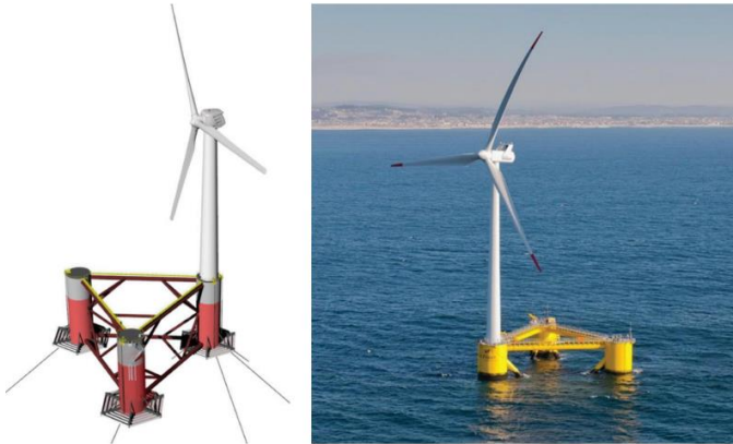
Figure 9. Semi-submersible type FOWT design & application [15]
