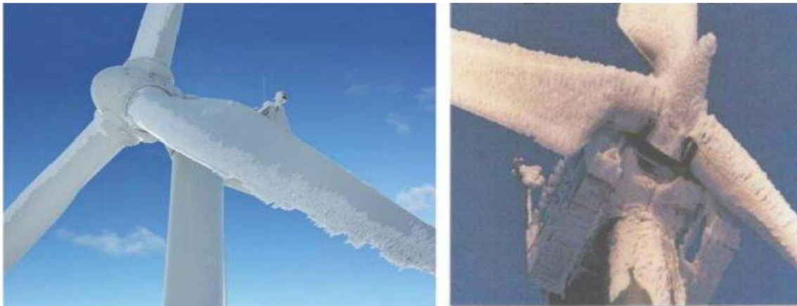
Figure 23. Atmospheric icing on wind turbine blades [42]
