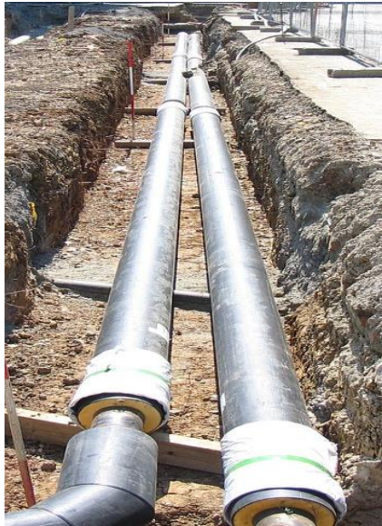
Figure 32 Trenched piping footage
