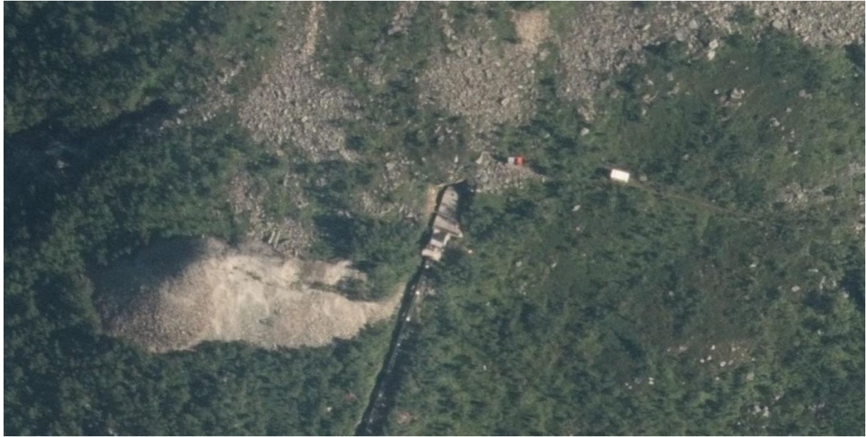
Figure 33 A screenshot aerial footage shows the area where the penstock becomes underground in Niingen mountain at coordinate (68.544481, 17.029082) [39]
