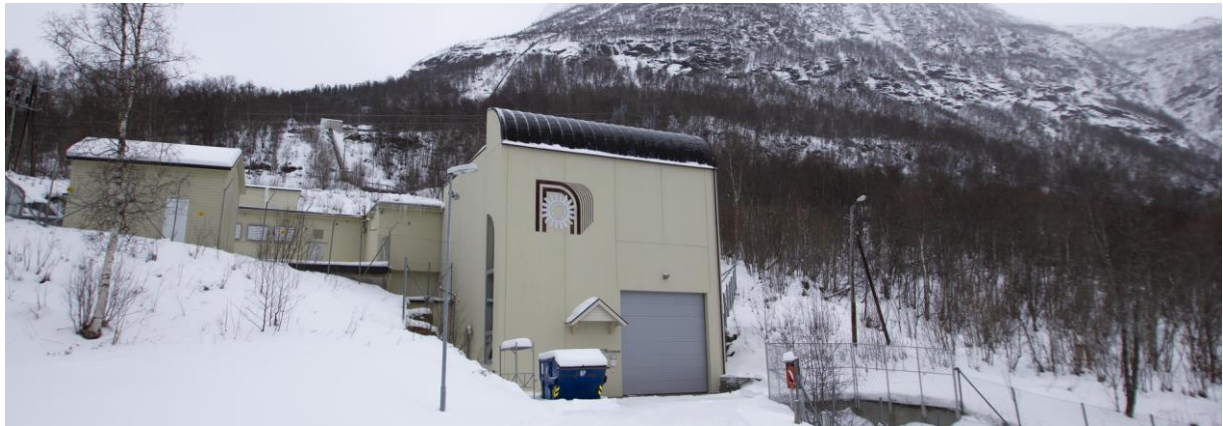
Figure 1 Niingen Power Plant [4]
