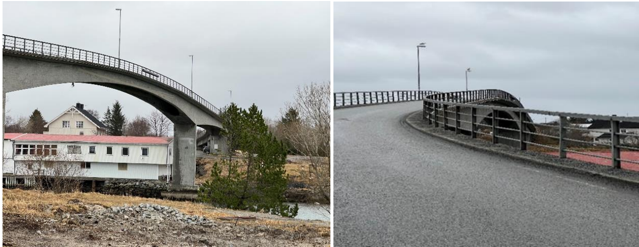
Figure 1: Overview of the Herøysund Bridge
