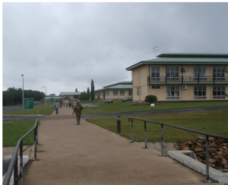
Figure 4: Volta Regional Hospital
