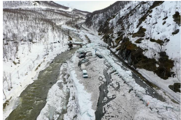
Figure 5: The slushflow travelled down an open and flowing river. The runout was several km down a gentle sloped river. Debris of ice and snow can be seen on the road and in a parking lot. Photo Trond Nilson
