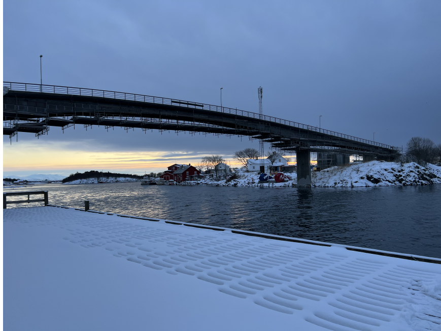
FIGURE 4. Herøysund Bridge located in Nordland, Norway
