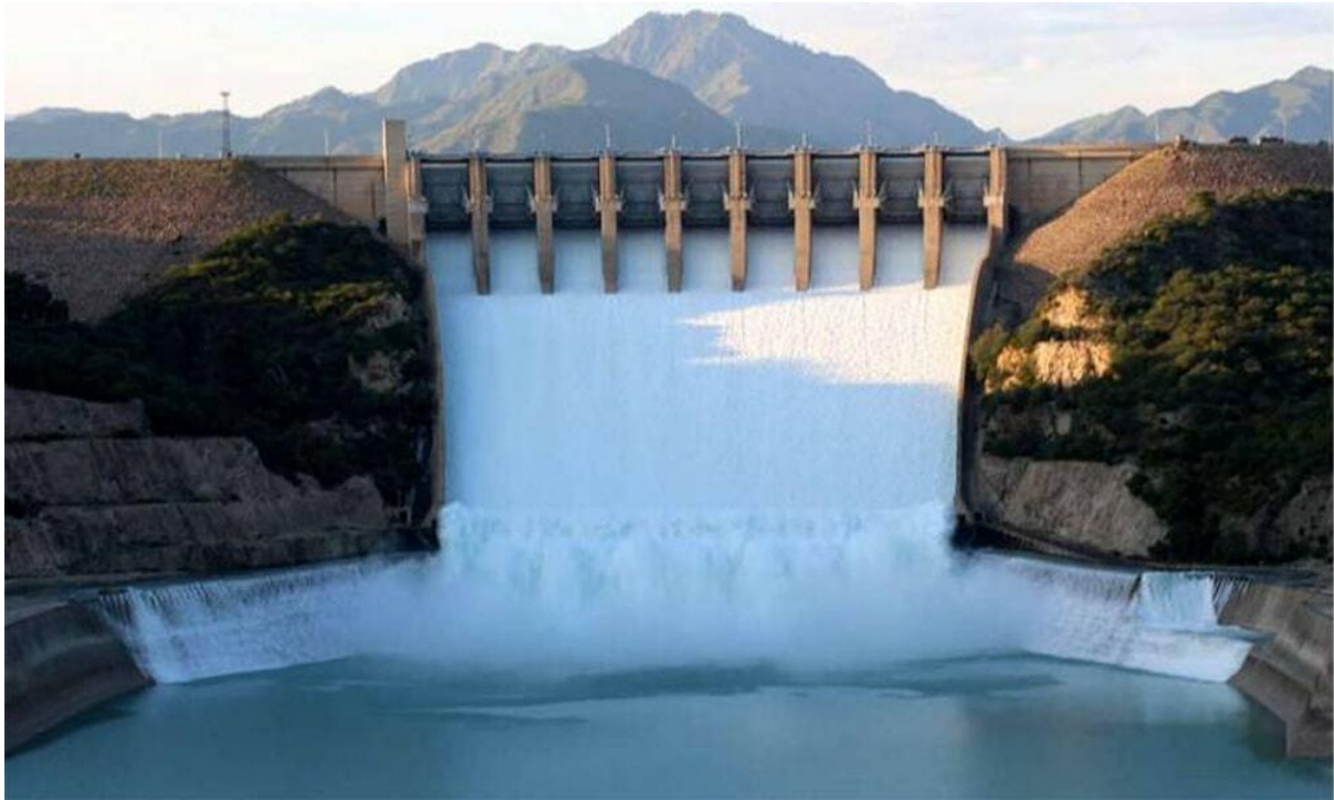
Fig. 5.1 shows Tarbela dam located in Tarbela, Haripur District , after spillways have been opened (Hamid Waleed) August 20, 2024
