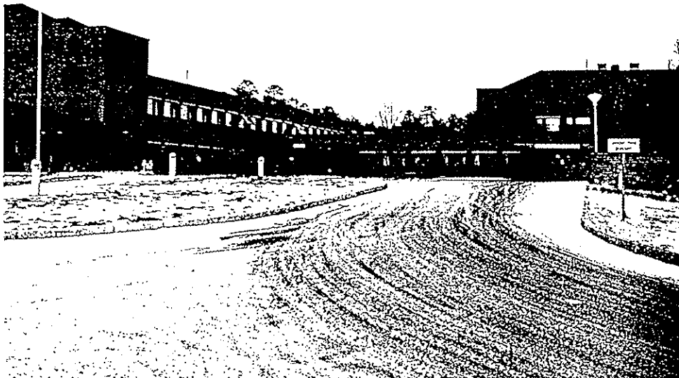
Modern health centre including GP hospital, Alta, 1997
