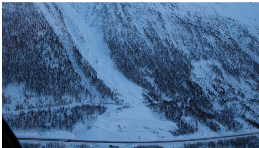
Figure 1.2: A large avalanche released by Staten Vegvesen is stopped by two avalanche meadows in Lavangsdalen, Troms. Foto: Statens Vegvesen
