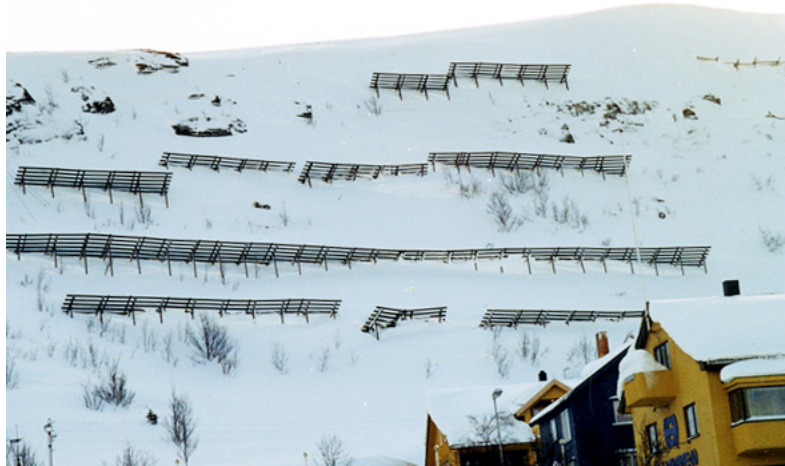
Figure 1.1: Avalanche fences installed above residences to stop avalanches from happening in Hammerfest, Finnmark. Foto: Statens Vegvesen
