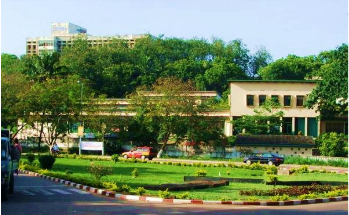
Figure 4: View of ENRH showing the OPD and the Tower building
