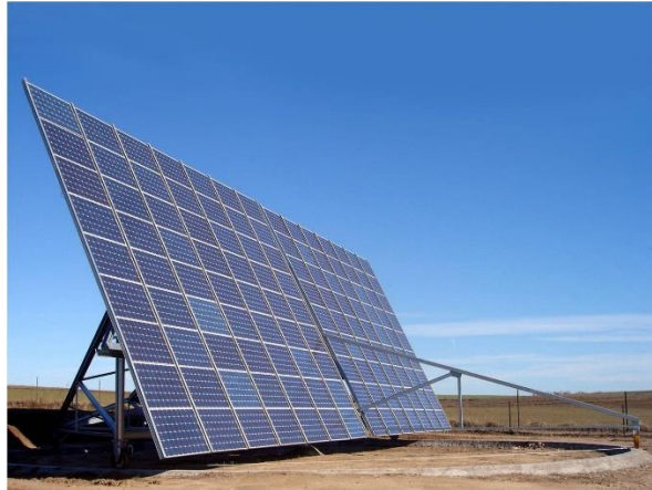
Figure 2.5.3 Azimuth-Altitude Dual-Axis Solar Tracker [28]
