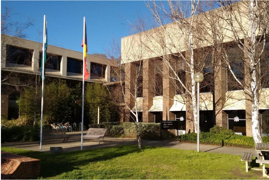
Figure 2: Entrance to the Tjabal Centre
