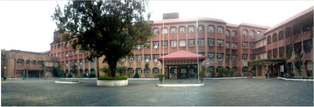
Figure 2: View of BPKIHS
