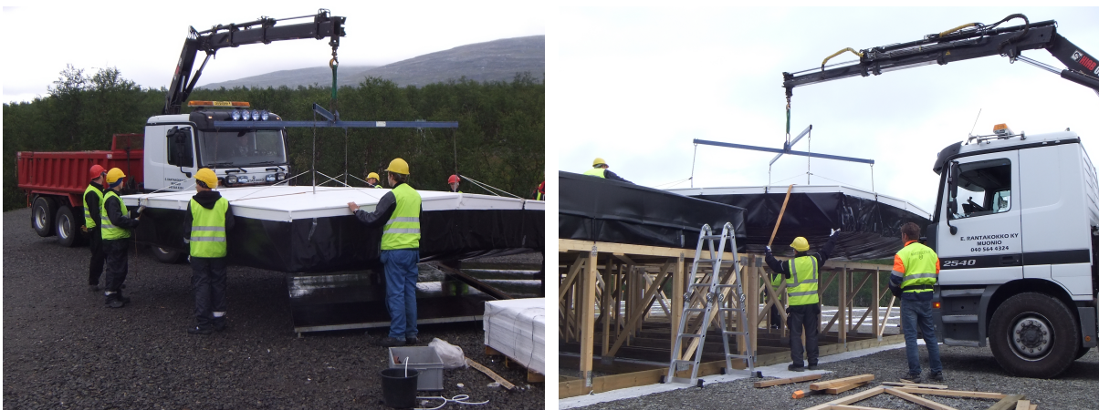
Figure E.29: Moving the partially-completed HBA tile from the unfolding station (left) to the final position on the relevant frameset (right).
