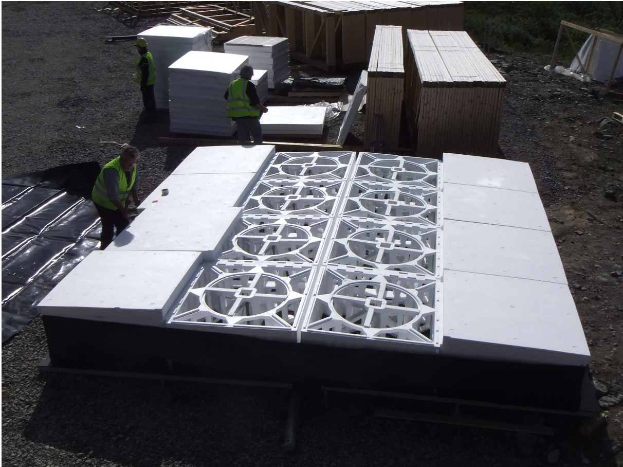
Figure E.28: A partially-fitted HBA tile on the unfolding station. The lifting/unfolding pin used to transport the tile out of storage is still below the tile in the gap between the platforms. The outer rows of lids have been fitted. Beyond the assembly area are stacks of lids and timber frames for the frameset construction. The tile cover can be partially seen on the left. It is not fitted until after the tile has been lifted into place.
