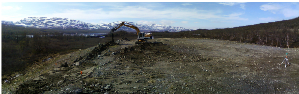
Figure E.13: Composite panorama, looking northwest across the site. Existing roadworks' spoil material was moved to provide a roughly-level working surface for the application of fine gravel.
