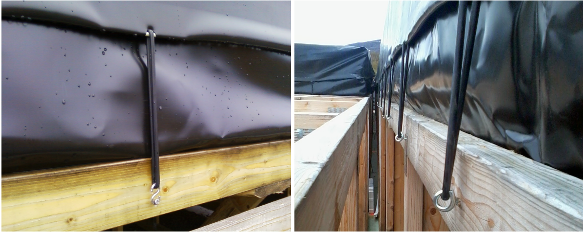
Figure E.31: Comparison of the two types of HBA cover securing arrangements. The left-hand image is the original design, with an S-hook attaching to a drywall screw. Note the top of the O-ring, where it connects to the white fibreglass rod embedded in the edge of the top-cover. The right-hand image is the new implementation, with the O-ring connecting directly to a pig-tail hook.
