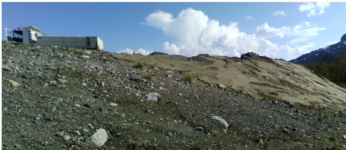
Figure E.14: Composite panorama, looking south at the development of the mound. The lighter, smoother area on the right is the new material. (See also Figure E.32.)
