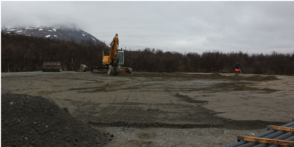
Figure E.41: LBA field groundworks. Image: Joonas Keskitalo, SGO.
