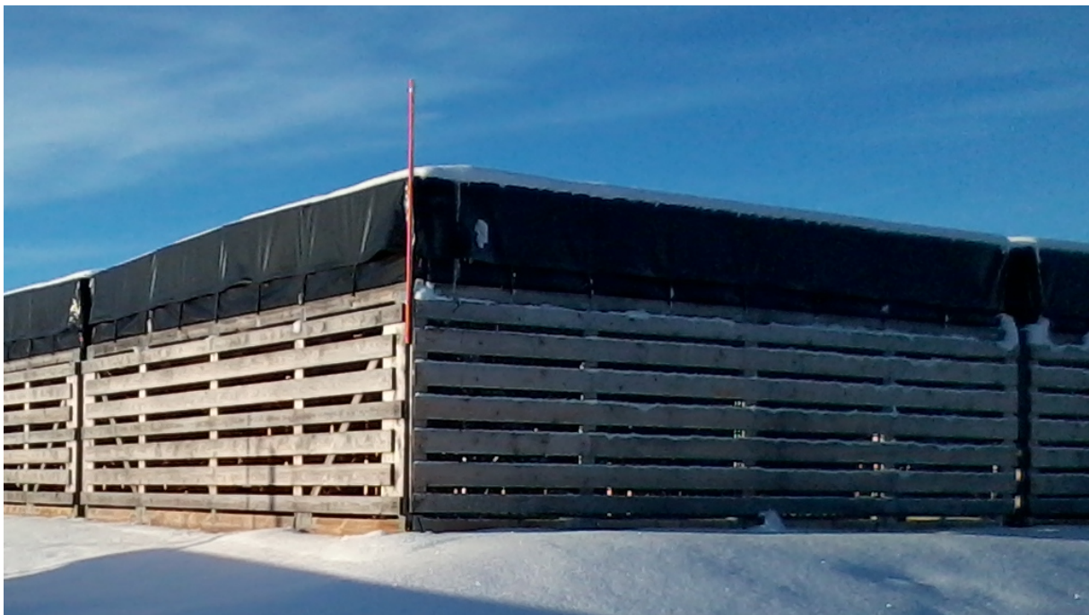
Figure 2.4: An example HBA tile (#H31). The top cover of the tile is anchored onto the supporting timber frameset, holding the tile in place. Each tile stands independently of neighbouring tiles.
