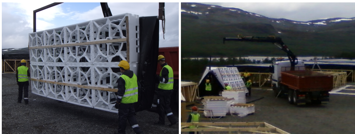
Figure E.26: Moving the tile from storage to the unfolding station (left) and then unfolding it as it is lowered into position there.
