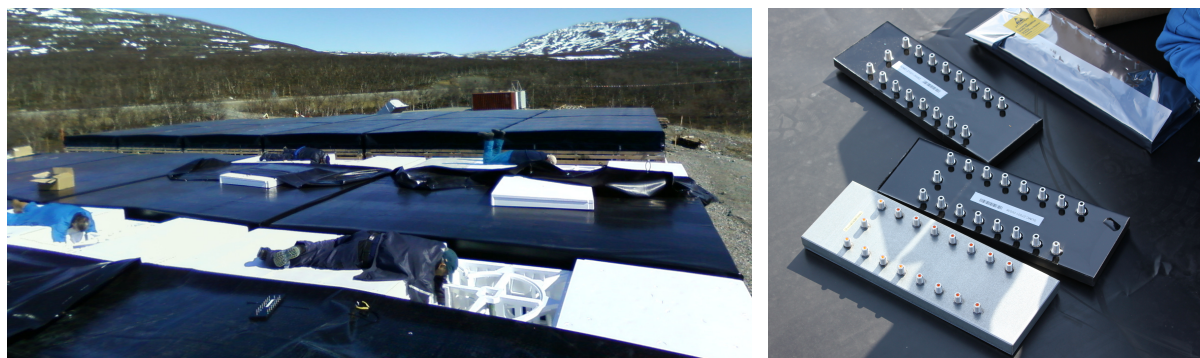
Figure E.38: Fitting summators into the HBA tiles (left). Examples of individual summators are shown (right), including both a light, sheet-metal Mark-I design and some dark, resin-filled Mark-II summators.
