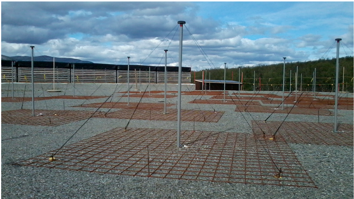
Figure 2.5: An example LBA aerial (#L35) in the foreground, amongst numerous others. The small structure with the sloped roof is the LBA array cable mausoleum (Appendix E.15) and the southeast edge of the HBA array is also visible.
