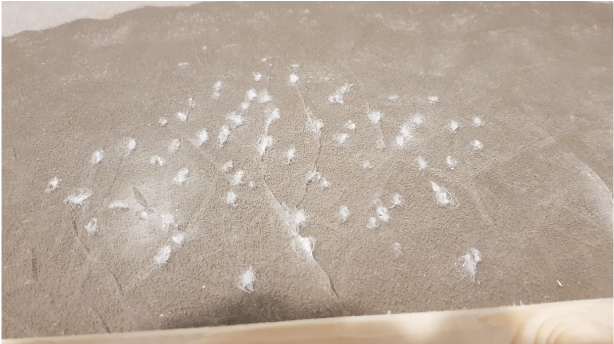
Figure 23: Ice removal from concrete
