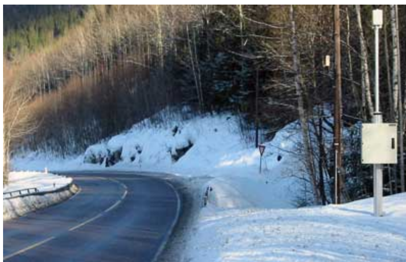
Figure 11: Example of Road weather station. ScanMatic
