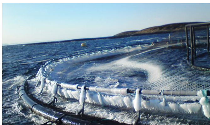
Figure 15: Image of a cage at a fish farm facility that is covered with ice during winter [75].
