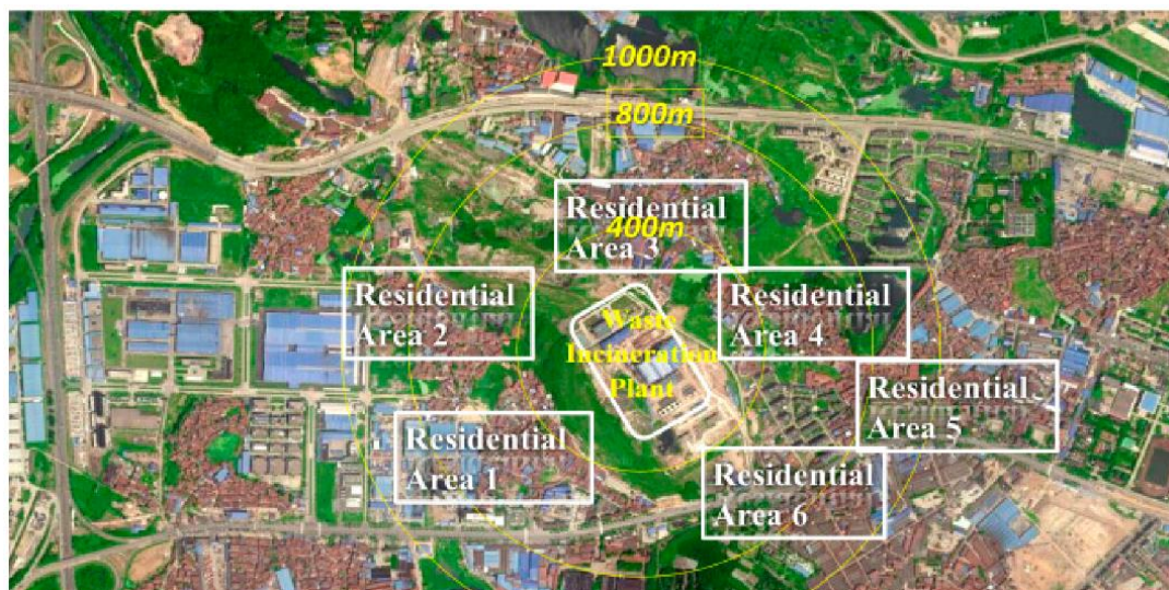
Figure 1-12 Location analysis of the impact of Guodingshan incineration plant on nearby residential areas (Hu et al., 2015).
