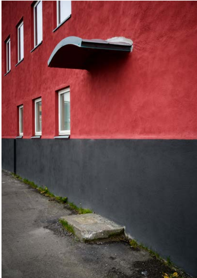
No entrance! Vardø Town Hall; an entrance was closed after renovation works. Photo: Farstadvoll
