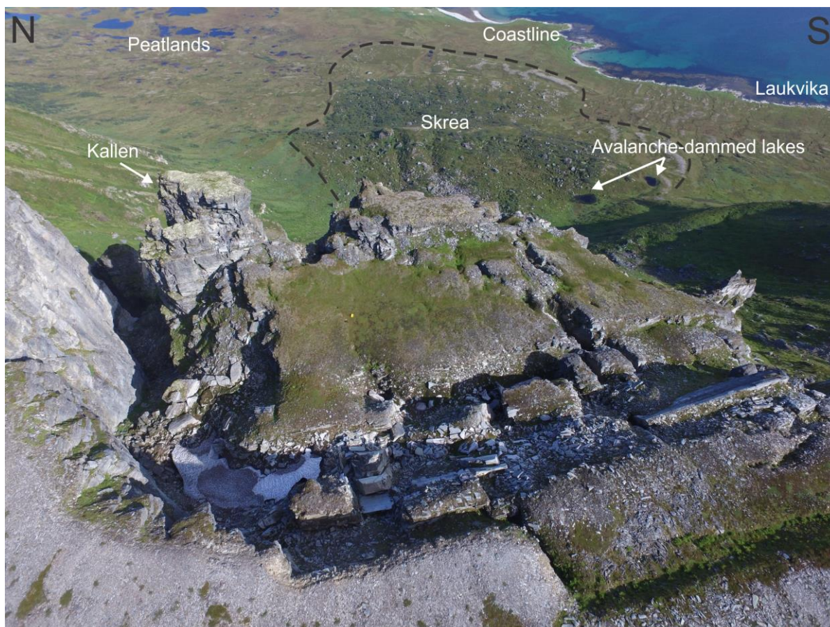
Figure 2: Drone photograph from August 2018 giving an overview of the study area. The avalanche-dammed lakes and the column "Kallen" are marked with arrows, while the rock avalanche deposits ("Skrea") are marked within the black stippled line.
