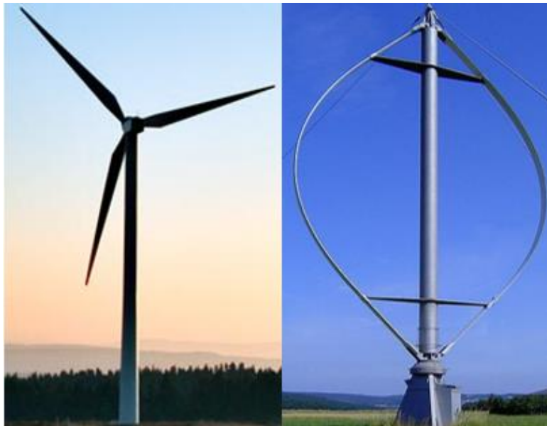
Figure 1: To the left a horizontal-axis wind turbine [42] and to the right a Darrieus vertical-axis wind turbine [43].
