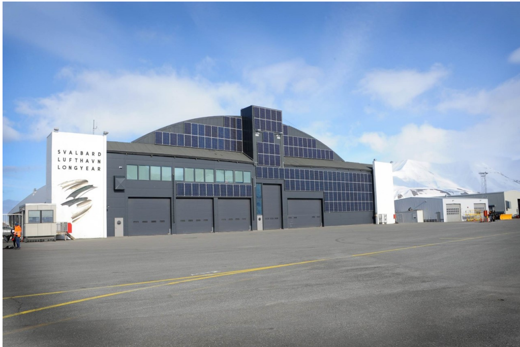
Figure 30: Modules on hangar.
