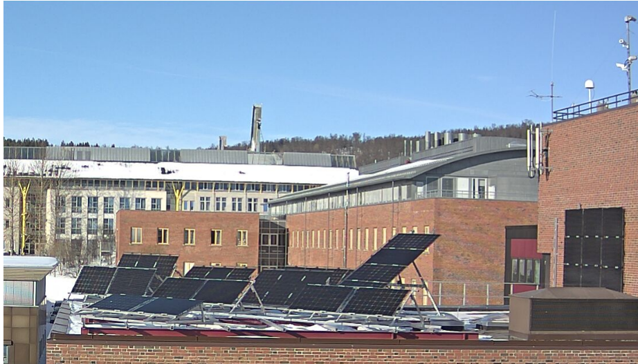
Figure 14: Solar energy system at UiT, campus Tromsø.
