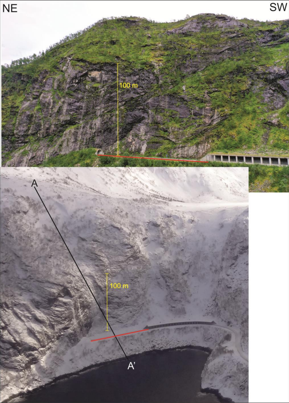
Figure 3. Drone photo and photo taken from helicopter of Svartholla during summer and winter, showing the research extent. The 100 meters stretch of road (red line) that is being investigated is situated between the Svartholla tunnel to the left and the rock shed to the right. Note the steep terrain that characterizes Svartholla, especially the 100 m high cliff above the road. Also note that the profile line (A-A') used for the slope profile shown in the next figure is marked. Photo 1: Linn Asplin, 2020. Photo 2: Andreas Persson, 2018.
