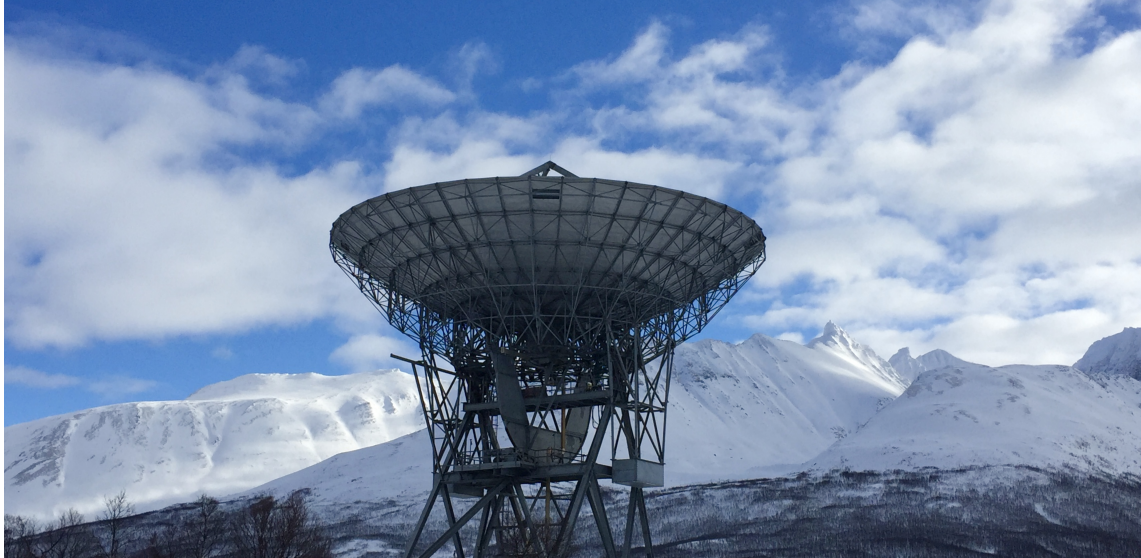
Figure 3.4: The 32-meter diameter dish of the EISCAT UHF radar in Ramfjormoen, Norway on a sunny winter day.
